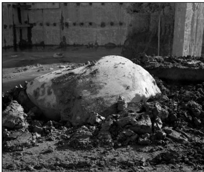
Casting Basin Excavation: Boulder found imbedded in the clay layer. (February 2, 1997), copyright Don Eyles.
